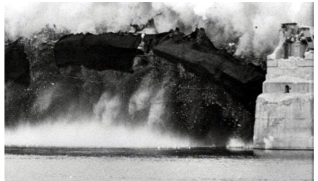
Bridge Demolition May 1996
